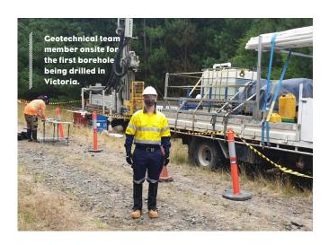
Ceotechnical investigations provide detailed information about soil conditions allowing engineers working on the project to design the cable system and converter station sites correctly.
