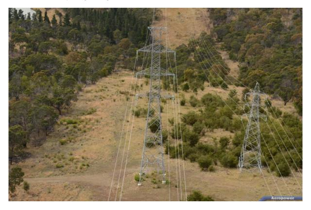
Plate 3-1 Typical double circuit 220 kV transmission tower adjacent to typical double circuit 110 kV transmission tower
